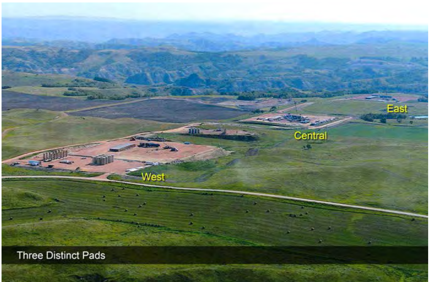
Aerial view of surface operations associated with the Hawkinson Project.
